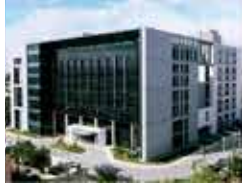
Taoyuan Technology Center (Green Building)
